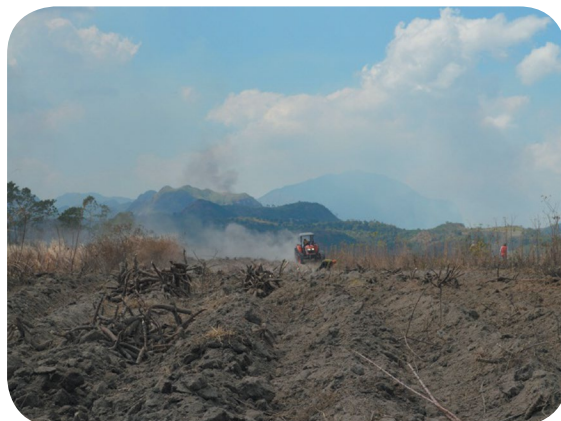
Terrain at test site during and after mechanical digging
